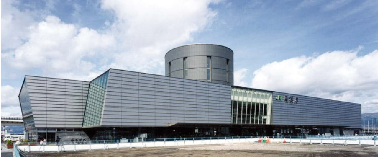
Photo. 1 Hakodate station of Japan Railway (Hakodate, Hokkaido). JR 函館駅(函館市)
